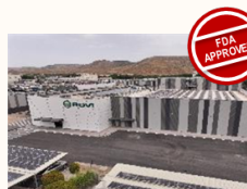
ROIS Alcalá de Henares Center of excellence for injectable packaging and assembly
